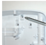
Multiple legacy wall fixings
